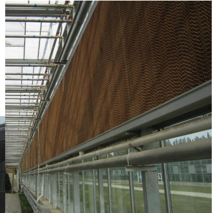
Evaporated pad wall
